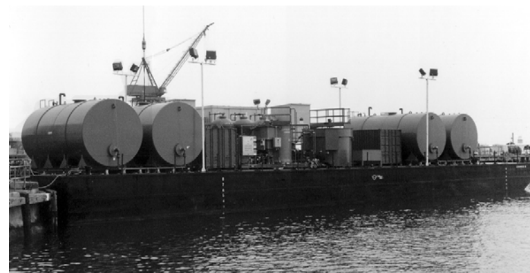
The TBT treatment plant resides on a barge that can be moved between dry docks as needed.
