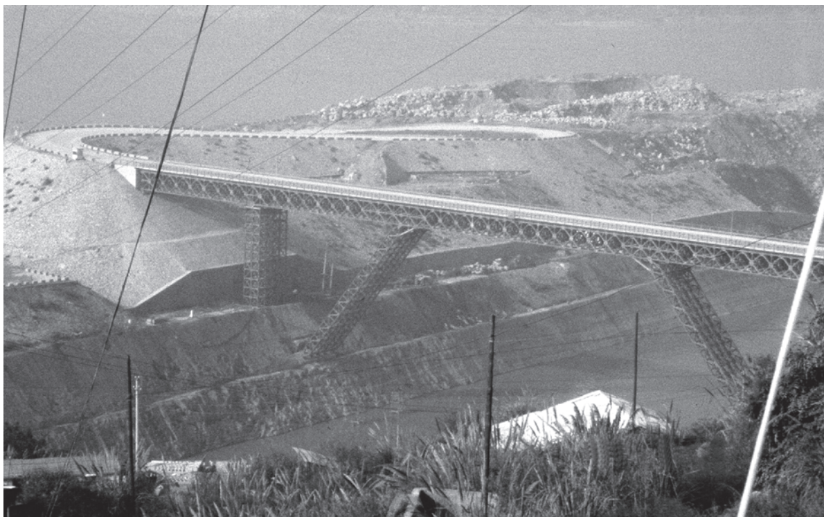
Construction on Three Gorges Dam.
