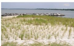
Hybrid living shorelines combine organic features with structures to support wide tidal marshes and beaches. Offshore breakwaters combine beach sand and dune plants with large structures that intercept incoming waves to support wide sand beaches. This approach is suitable for higher energy beach shorelines. Research has shown that hybrid living shorelines and the habitats they support provide cleaner water, economic gains, and cultural traditions as ecosystem service benefits.
