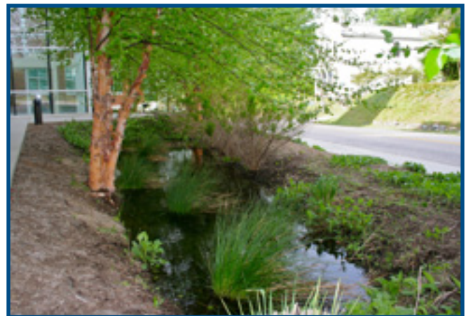
A rain garden in front of Andrews Hall helps collect and manage the building's stormwater runoff and air-conditioning condensate.
