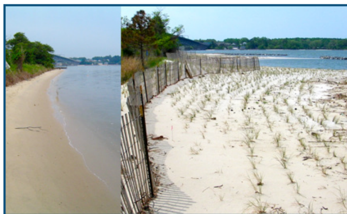
Before & After: These before and after pictures of a VIMS beach show how emplacement of a breakwater provides a wider buffer against wave energy as well as habitat for native plants. Photos courtesy Scott Hardaway.
