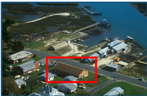
Seaside Hall: The fire destroyed Seaside Hall, the building outlined in red.
