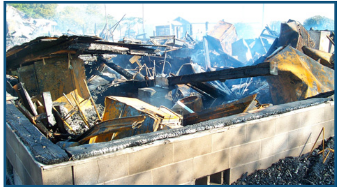
Wreckage: The fire completely destroyed the building's contents.
