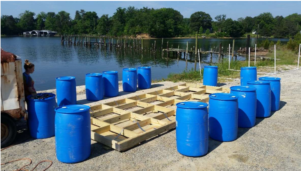
Barge has been flipped.
