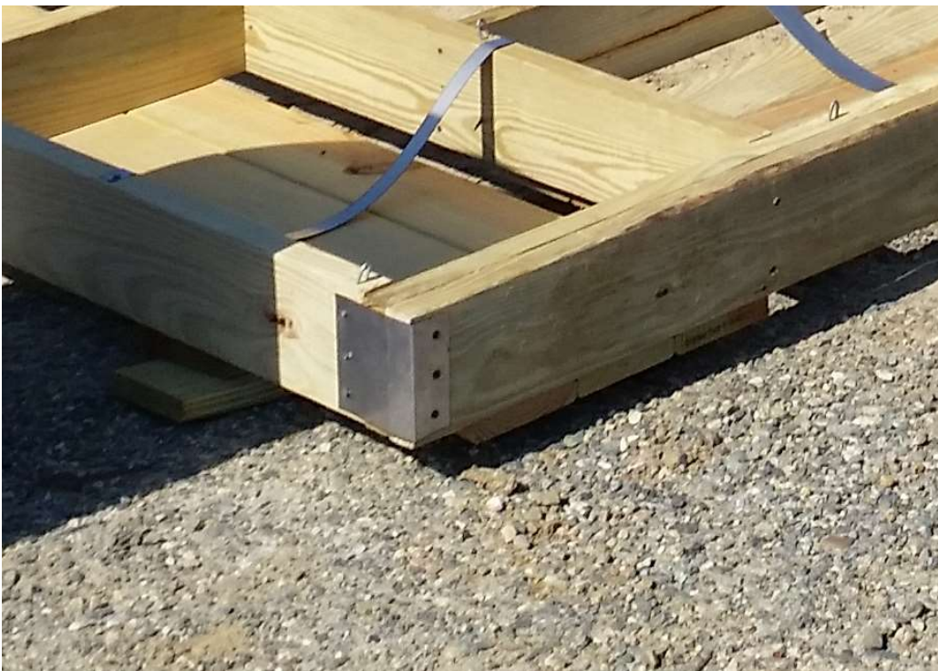
Caption: Again, note the barrel strap that will be on the top of the barrel and the metal plate around the corner. Both of these keep the stress of the weight from popping the screws.
