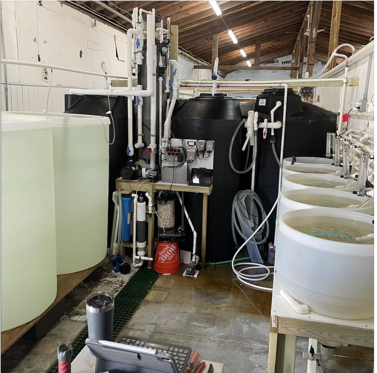
Figure 3: Photo of complete pilot scale system.
