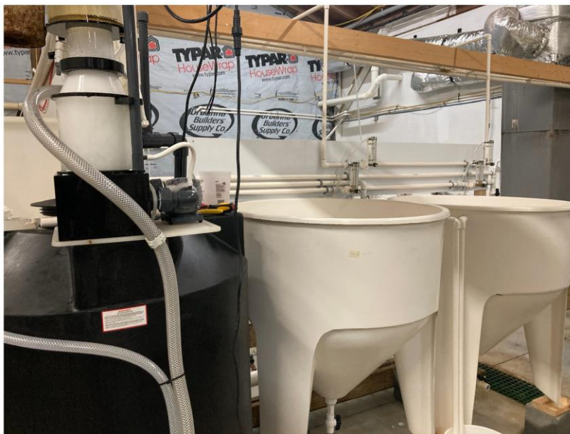
Figure 1: Preliminary small-scale RAS at OSH in 2020. The bioreactor/filter is the black tank to the left.
