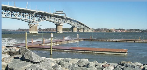
The docking facilities at Riverwalk Landing were funded in part by a Tier 2 – National Boating Infrastructure Grant. Photo by Preston Smith.
