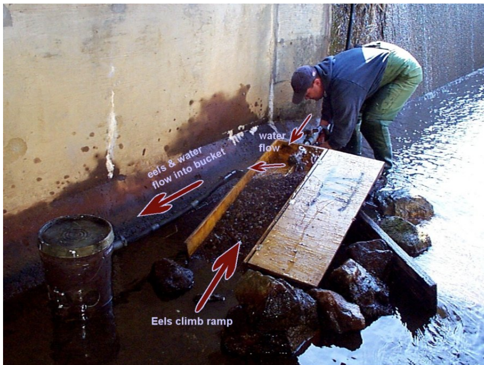
Figure 2. The Irish ramp at Gardy's Millpond showing its configuration. The arrows indicate the flow of water as well as eels.
