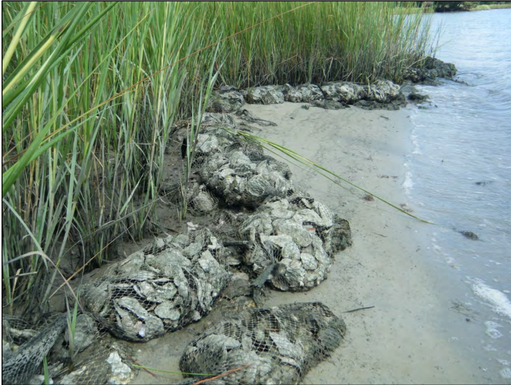
Oyster shell bags placed along eroding marsh edge
