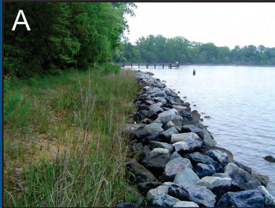
Sill at St. Mary's City A) five years after construction (9 May 2007), B) 16 years after construction (15 Aug 2018). Phragmites has colonized behind the structures.
