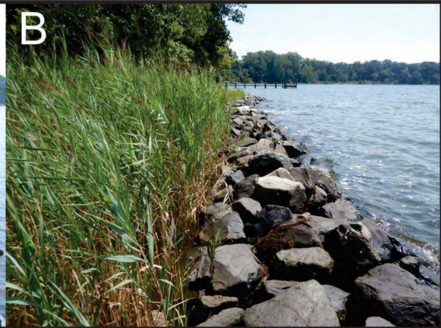
Sill at St. Mary's City A) five years after construction (9 May 2007), B) 16 years after construction (15 Aug 2018). Phragmites has colonized behind the structures.
